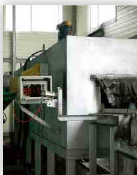
열처리 제어냉각 HEAT TREATMENT & CONTROL COOLING
